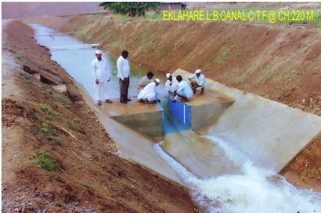
Cut throat flume arrangement for Eklahare Minor Irrigation Tank, Taluka Dindori, District Nashik.
