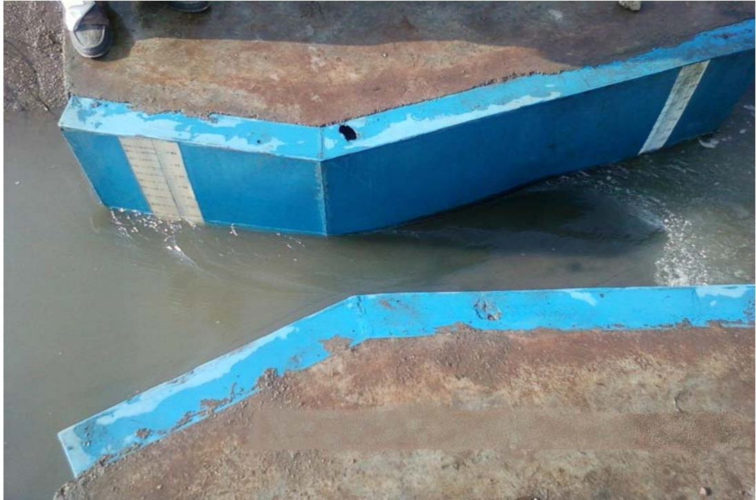
Cut throat flume arrangement for Telhara Minor Irrigation Tank, Taluka Chikhali, District Buldhana.
